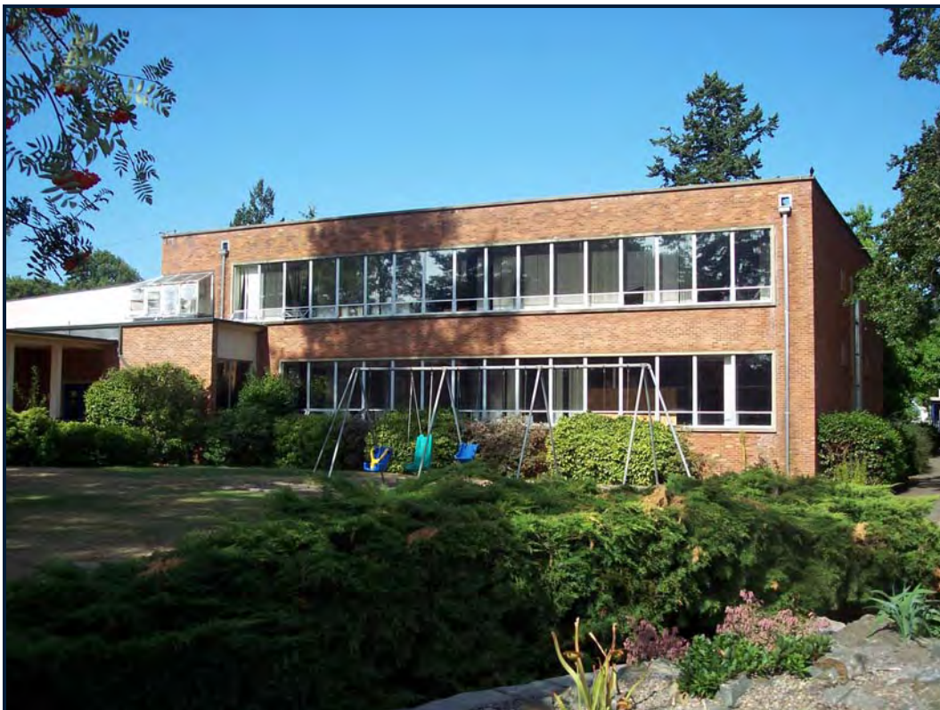
Looking west to the north wing of the school building.
