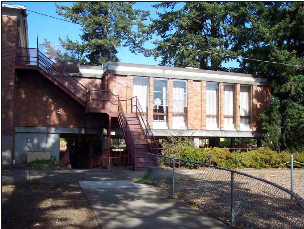
Dorm Building (Bracher Lounge – added 1966).
