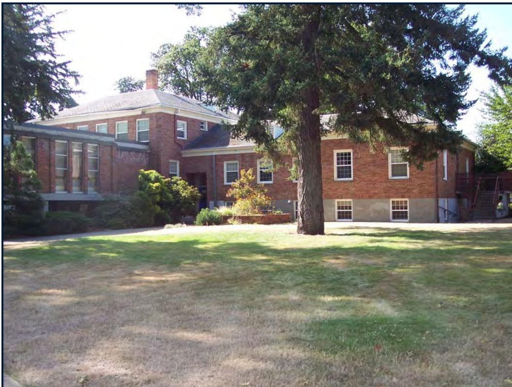
Looking south to dormitory.
