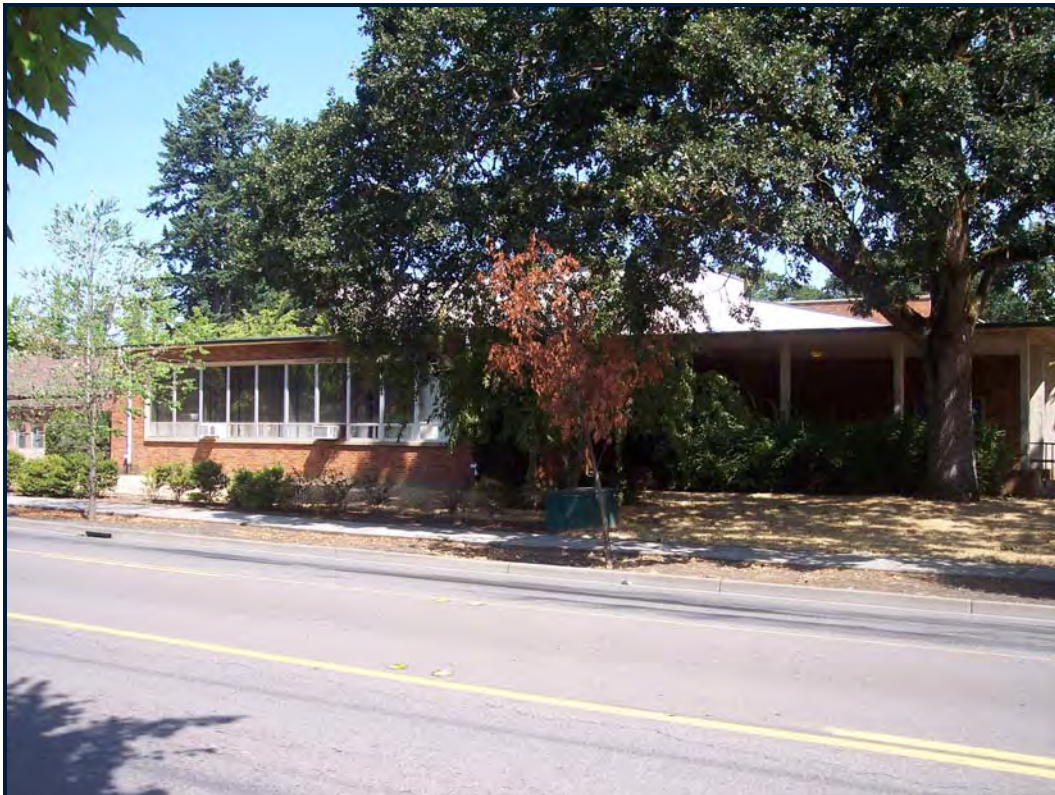
Looking north to School Building.
